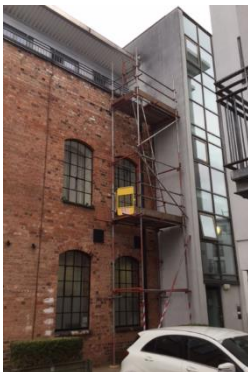
K Block - Scaffolding
