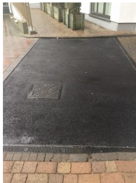
Car Park Entrance Current Finish
